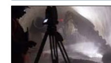
On the cover: A road-header at point 5 in August, preparing for the high-luminosity LHC upgrade. (M.Brice/CERN.) 26
