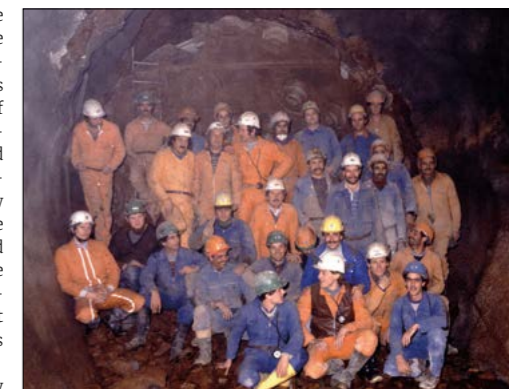
Heroic The LEP tunneling crew in January 1987 having completed the arc from point 2 to point 3 with only 1 cm of difference.
